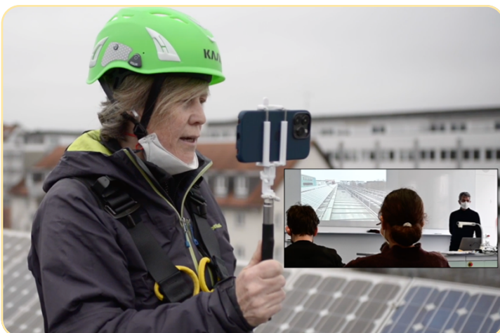
Christina from SOFS, livestreaming to a class while doing an annual inspection of the solar panels
